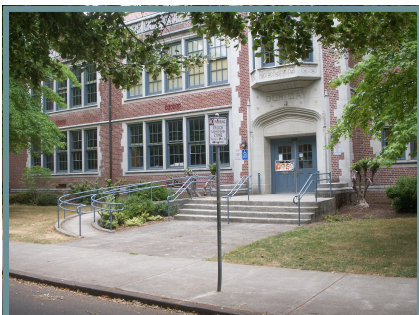
Compliant ramp/stairs with handrails
